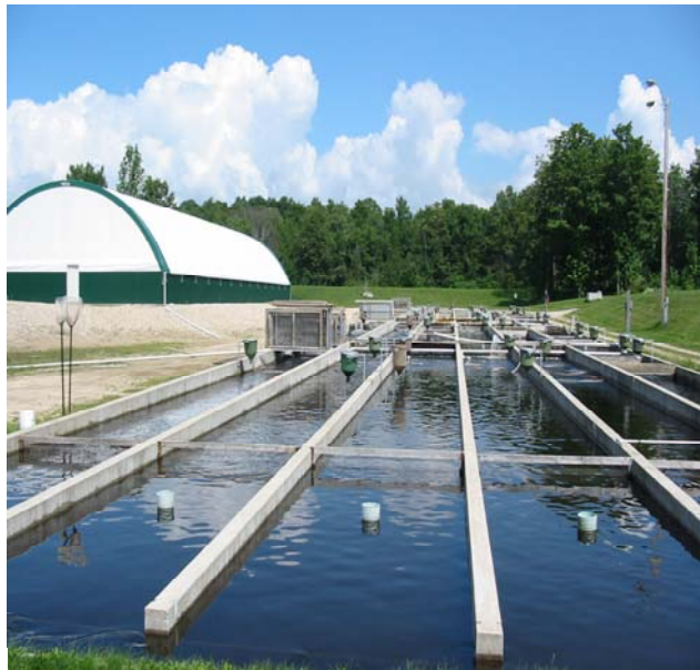
Land-based trout production facility showing concrete raceways with “in-tank” settling zones.
