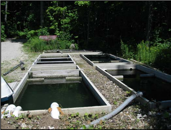
Small clarifier system constructed from pre-cast concrete septic tanks.
