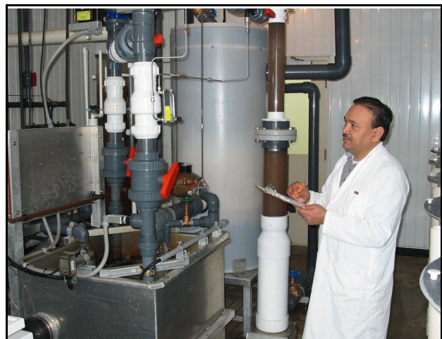
Recording oxygen injection levels.
