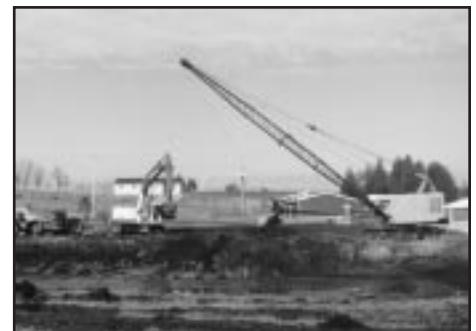
Pond construction on a natural watercourse
