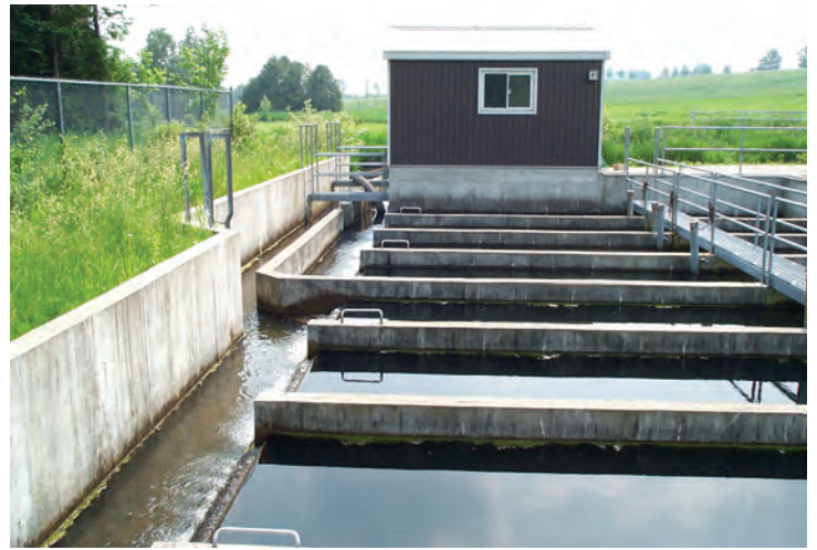
Figure 7. Solids require removal before water is discharged
