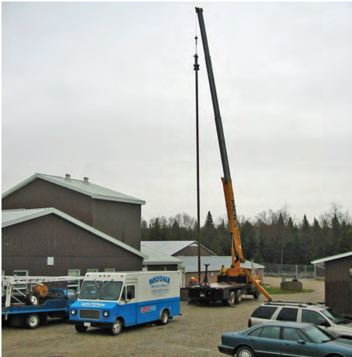
Figure 6. Well pump installation
